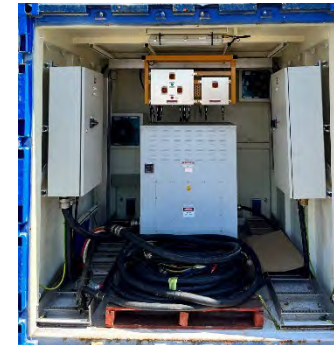
480V TO 690V STEP-UP TRANSFORMER
