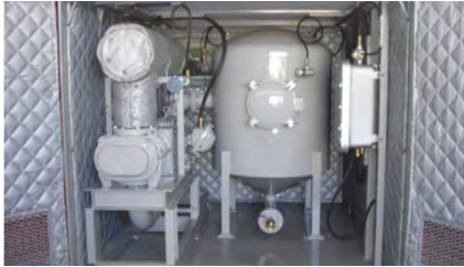
CONTAINERISED (10FT) VACUUM SYSTEM RIG-VAC RV-50HP
