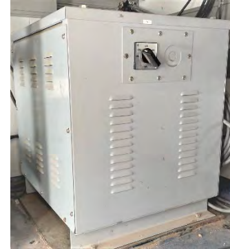
480V TO 690V STEP-UP TRANSFORMER
