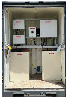
480V TO 240/220V DUAL TRANSFORMER
