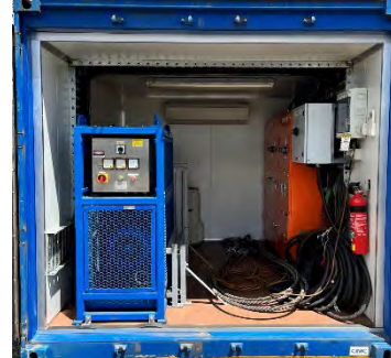
600V TO 480V TRANSFORMER AND POWER LINEATOR
